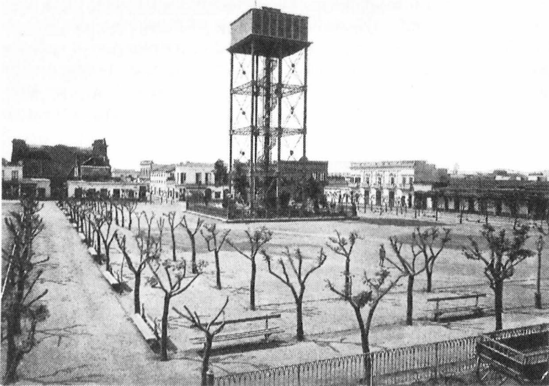
Figure 9.1 (a) Water cart filled in the River Plate, (b) Filtered water tank and water pump station in (then) Plaza Lorea, (c) First drinking water plant in (then) Low Recoleta, inaugurated in 1874 and enlarged in 1878. In the photo, the extension is almost finished, (d) Designed in 1877 and completed in 1894 with local and imported materials, the French renaissance Palacio de Aguas Corrientes (Palace of Flowing Waters) is both an example of turn-of-the-century eclectic architecture and an evidence of the cultural relevance drinking water had in the making of modern Buenos Aires.
